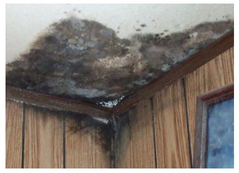
A roof leak that resulted in costly damage to the home
