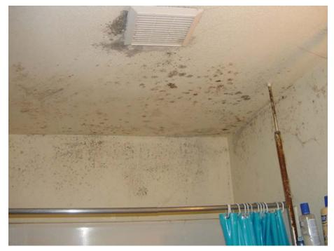
Broken fan and moldy condition that should be reported and repaired
