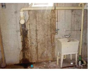
Water from a window and plumbing leak
