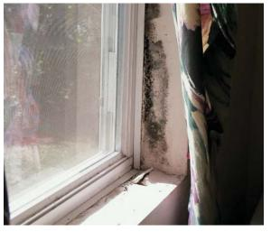
Mold damage from leaks at the window
