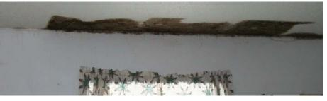
Mold caused by too little insulation or wind blowing the insulation away
