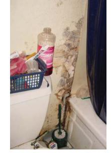
Mold and wall damage from water splashing outside the tub
