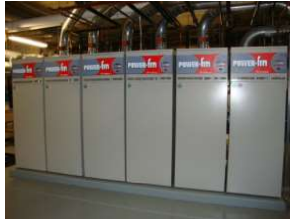
New Boiler Installation
