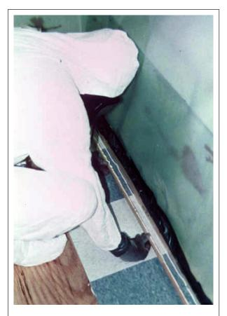
FIGURE 13.1 Encapsulating a floor with vinyl tiles
