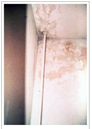
FIGURE 13.2 Deteriorated paint on surfaces that are unsuitable for encapsulation
