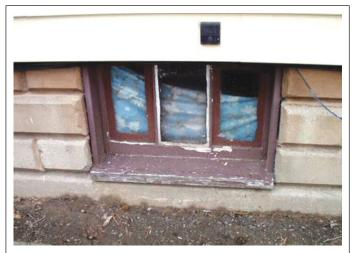
FIGURE 6.3 An area of bare soil beneath a window with deteriorated paint.
