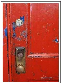
FIGURE 1.3 Paint deterioration.
