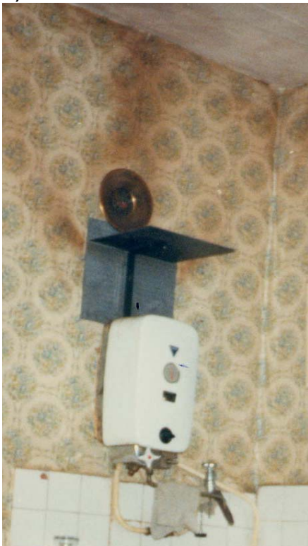
A) Gas instantaneous water heater
