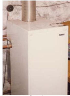
Gas-fired boiler
