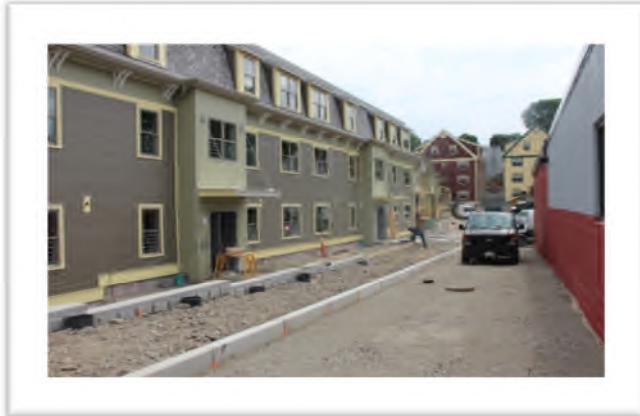
Construction underway at Quincy Heights, Boston
