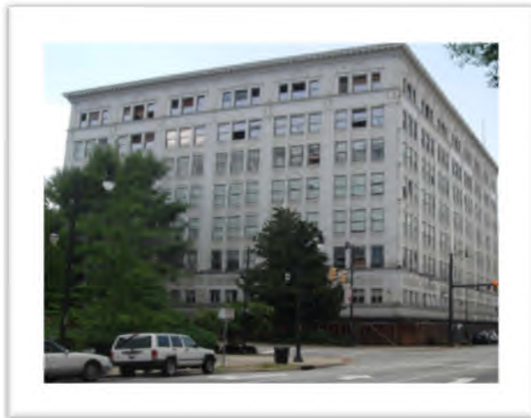
The historic Pizitz Building before renovation
