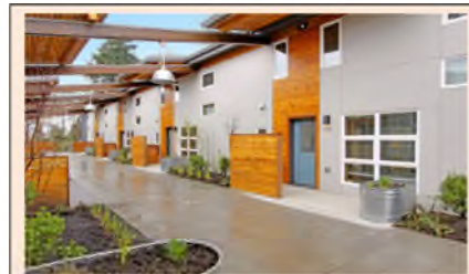
Near Tacoma, Washington and ancestral fishing grounds in Commencement Bay, the Puyallup Tribal Housing Authority is developing the NE Longhouse, a new, 20-unit housing complex with HUD funding provided under the Native American Housing and Self Determination Act and the American Recovery and Reinvestment Act. The U.S. Green Building Council certified the first phase of the NE Longhouse as LEED-Platinum, and selected the development as the Council’s 2012 LEED for Homes Project of the Year.
