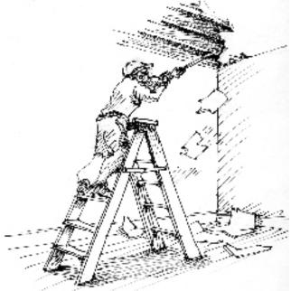
Work from a ladder so the ceiling can be pulled down in front of you. Use a tall enough ladder so you don't need your hips to be above the top of ladder. Never set the ladder on rubbish.
