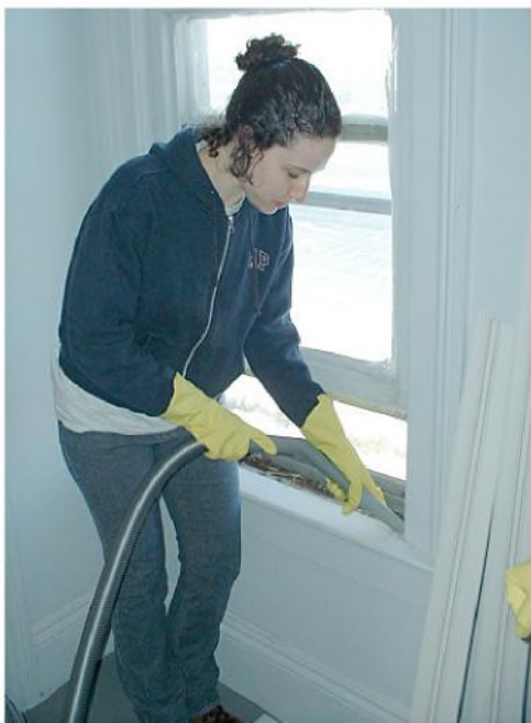
FIGURE 8.17 Pre-cleaning window with HEPA vacuum.
