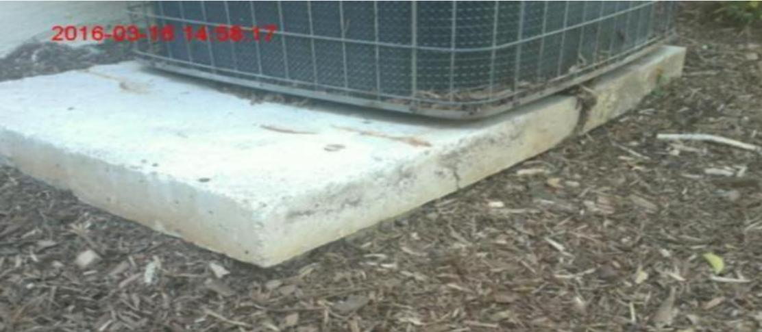
Often inspectors record a defect for erosion because the area under a tree or path that residence use does not have grass growing on it. This is not correct. Erosion shall be evaluated only if there is evidence of displaced soil.
