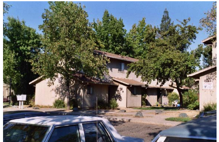
6250 Mariposa Ave., Sacramento: Pre-Modernization
