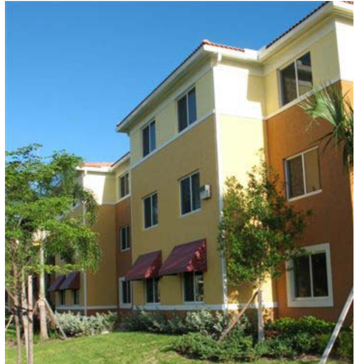
Tallman Pines: the first affordable housing in the state of Florida to earn the LEED Silver rating
