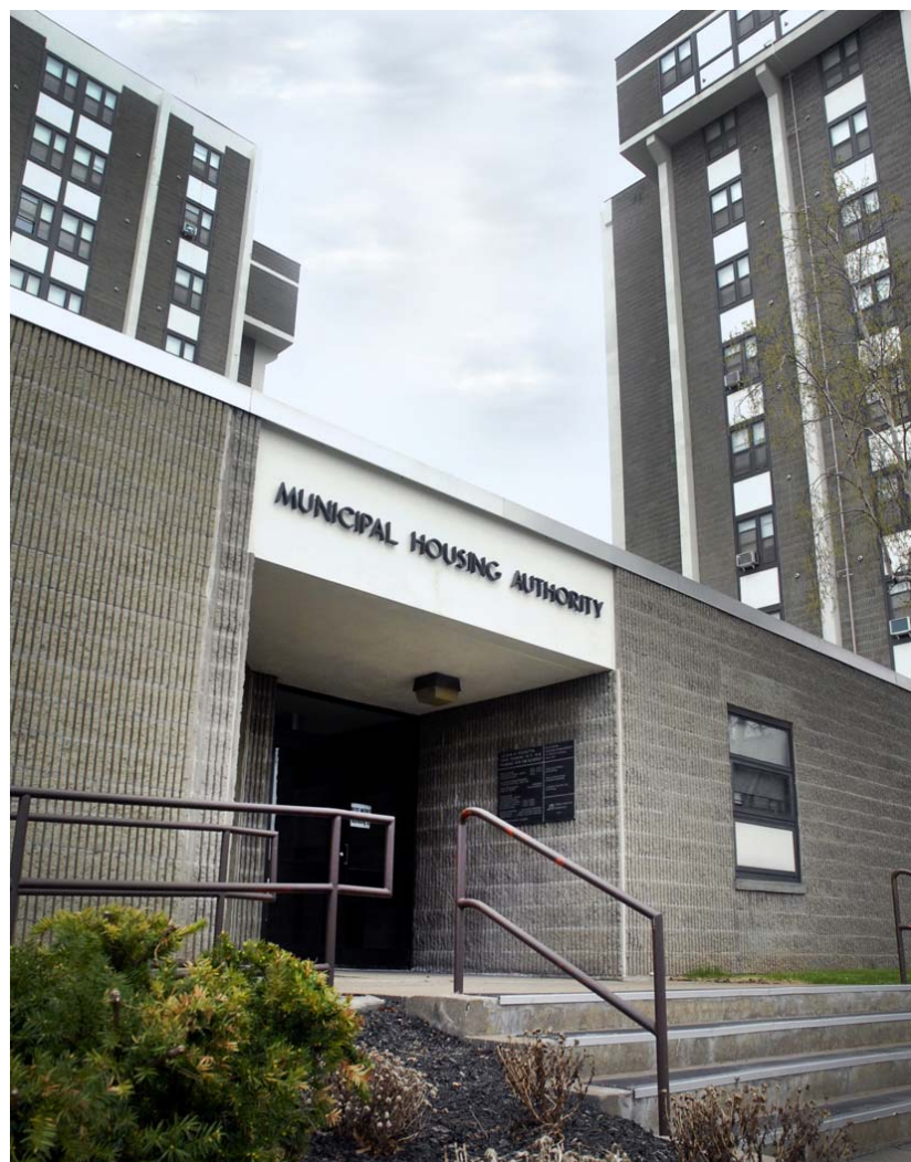
Central Office Cost Center, with the Perretta Towers 108 units of senior housing in the background. Photo by Pamela Jardieu
