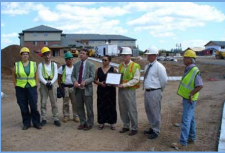
Award Presentation with Step-Up apprentices, Building Trades Council, Contractor, and HRA representatives (Photo: HRA)
