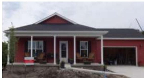
Picture 8- Homeownership under Construction
