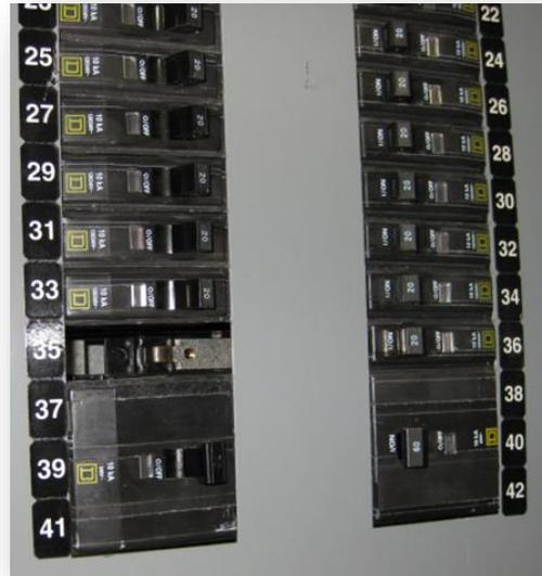
Electrical conductor is not enclosed or properly insulated (e.g., damaged sheathing, open port, missing knockout, missing outlet or switch cover, missing breaker or fuse, or missing lightbulb).
