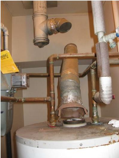
Chimney or flue piping is blocked, misaligned, or missing (i.e., evidence of prior installation, but now not present or is incomplete).
