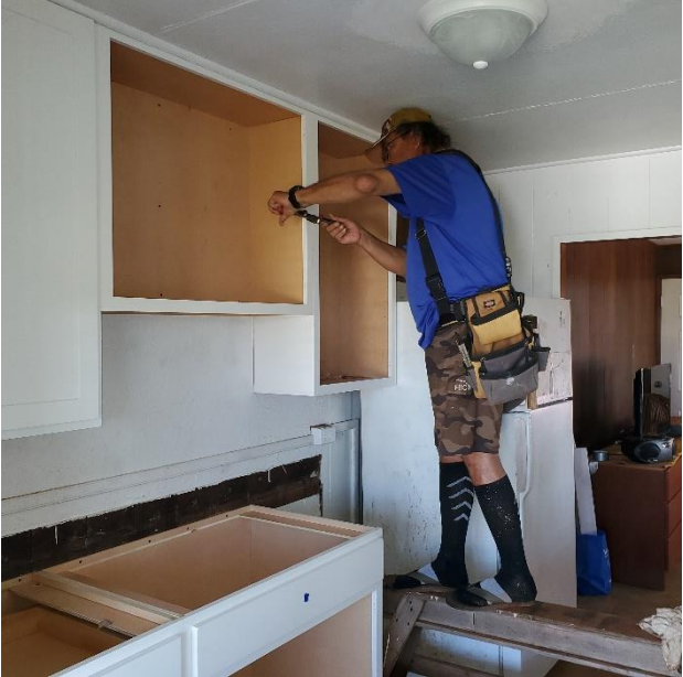
Figures 5 and 6: Home rehabilitation work in progress to replace kitchen cabinets, sink, and countertops
