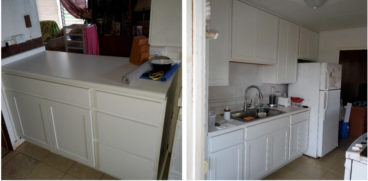
Figures 7 and 8: Kitchen rehabilitation work completed
