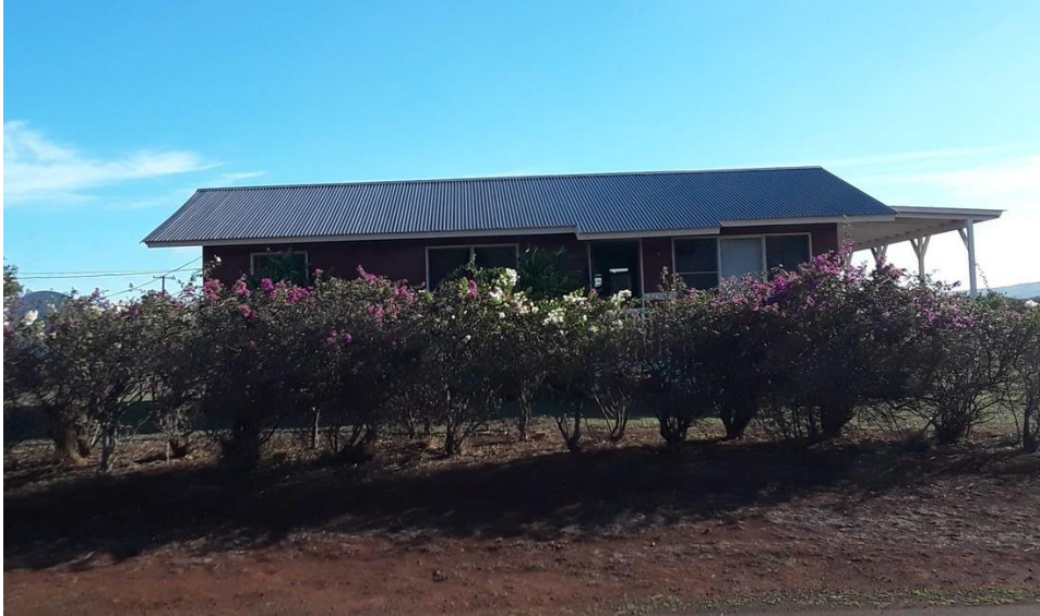
Figure 4: This home rehabilitation included replacing the roof
