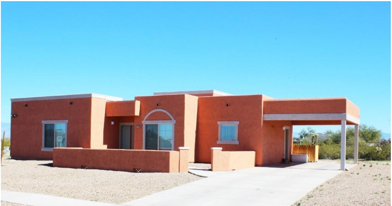
Figure 8: New Tohono O'odham home completed in 2020.
