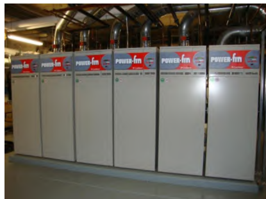
New Boiler Installation
