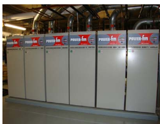
New Boiler Installation
