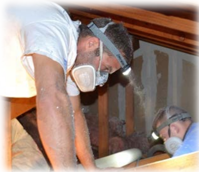
Crews blow in cellulose attic insulation at MPHA's Glendale Townhomes, through a partnership with Sustainable Resources Center (SRC) and CenterPoint Energy.
