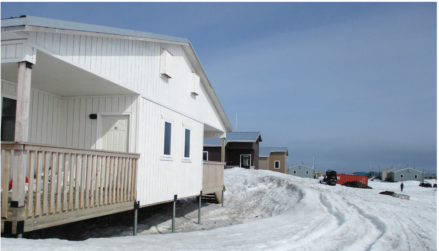
Helical piers stabilize the structure in this climate where a traditional foundation is not possible.
