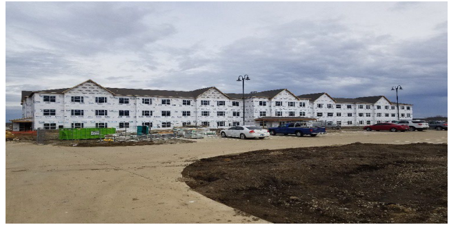
Picture 11 - Haven Court Under Construction
