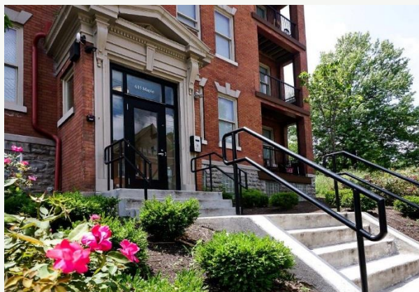
Figure 1: One of the formerly distressed target properties, after extensive rehabilitation
