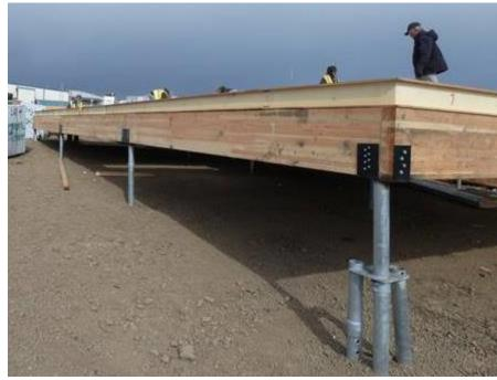
Monolithic pad built to prevent sluffing.
