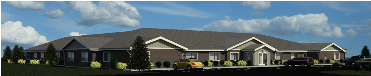
This is a picture of the completed Bridgeway Community Housing development.
