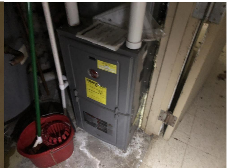
Gas fired water heater and Gas fired furnace (interior utility room)
