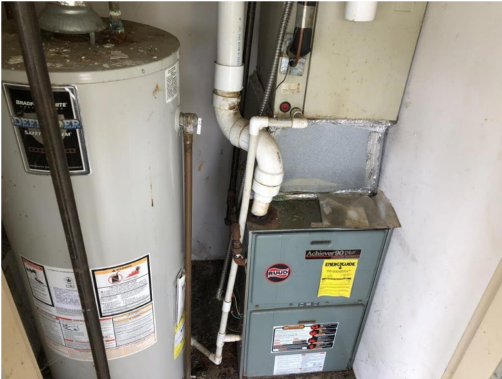
Gas fired water heater and furnace (exterior facing utility room)
