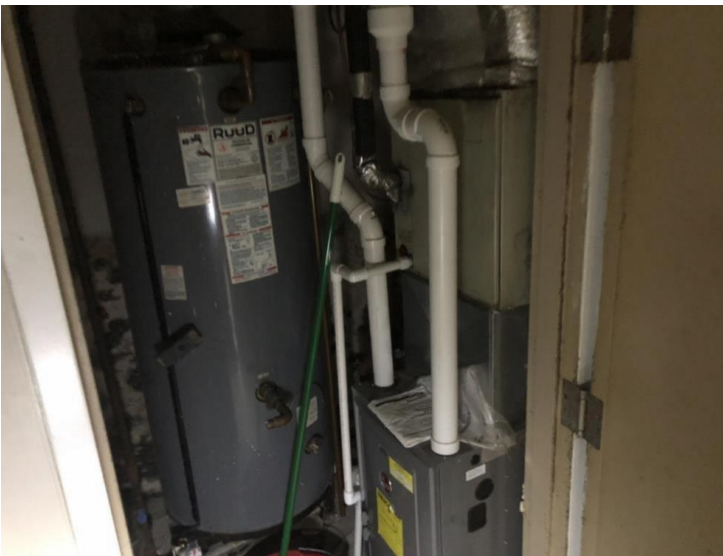
Gas fired water heater and Gas fired furnace (interior utility room)
