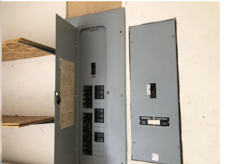
Building Breaker Panel
