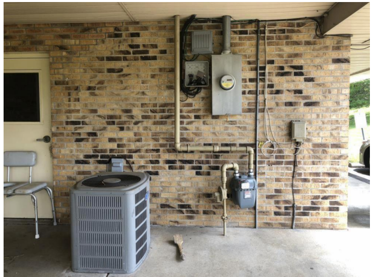
HVAC-Pad mounted condenser 1 and condenser 2; Electric & Gas Meters
