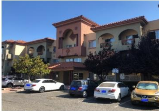
Photo 1. Front Elevation, SW View
