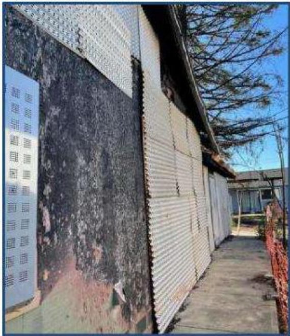
West Side of Building Damage
