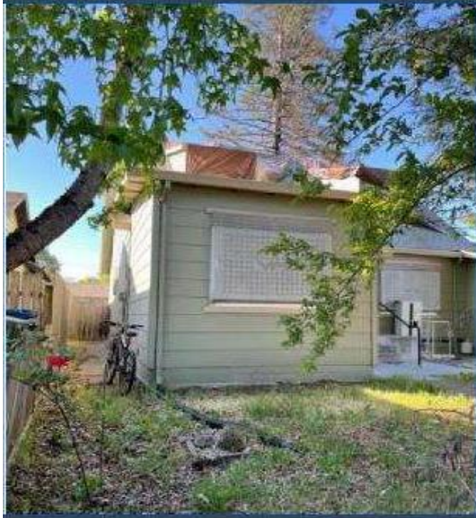
East Side of Building
