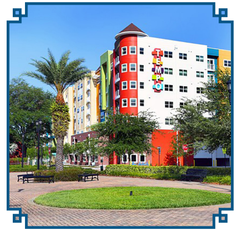
The Tempo at Encore, Tampa Housing Authority
