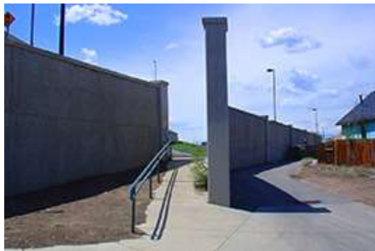
Noise Abatement and Control
