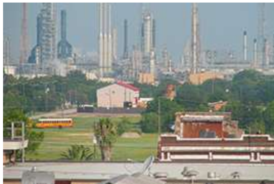
Explosive and Flammable Facilities
