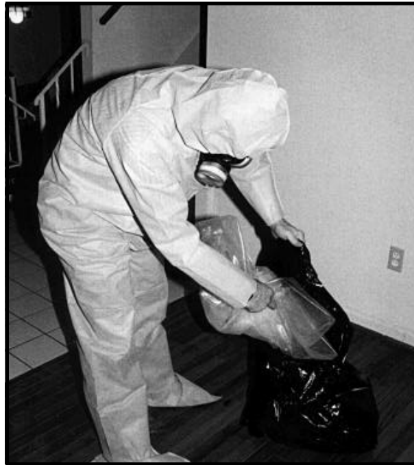
Figure 14.8c Dispose of Plastic Sheeting in a Plastic Trash Bag.
