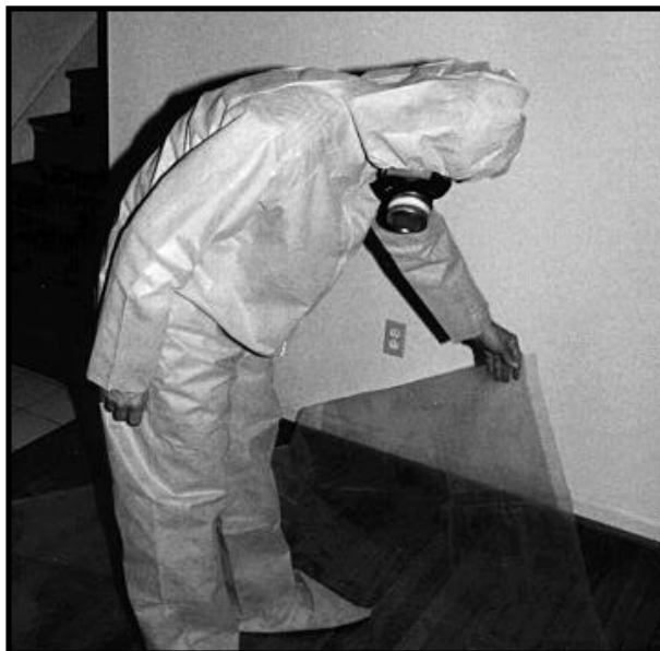
Figure 14.8a Pick Up Corners of Plastic Sheeting.
