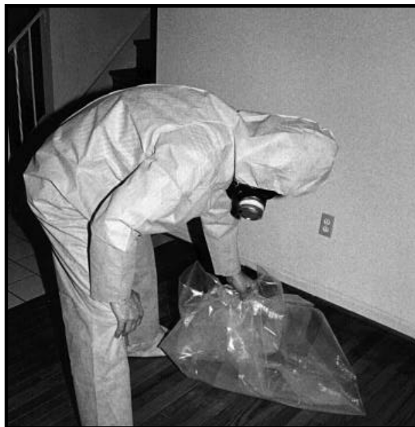
Figure 14.8b Fold Plastic Inward.
