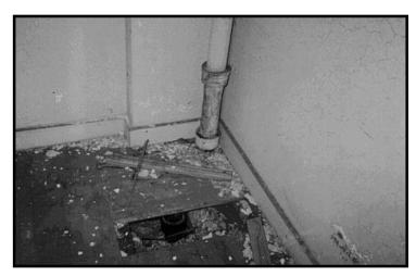
Figure 8.2 Area Should Be Precleaned and Structural Deficiencies in Flooring Repaired Before Lead Hazard Control Begins.
