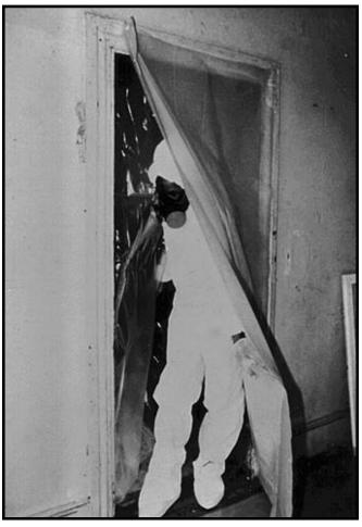
Figure 8.6 Install a Simple Airlock Over a Doorway to Minimize Lead Dust Migration.
