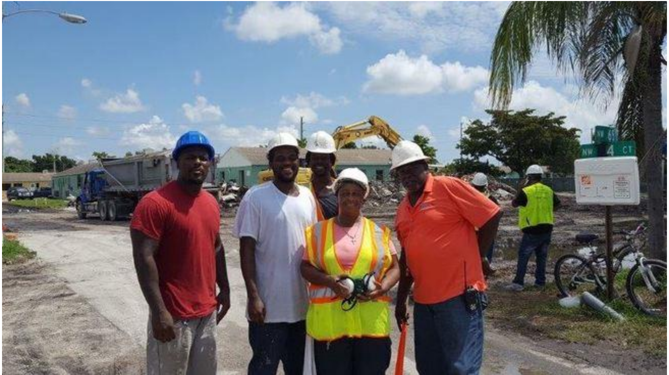
Photo (left to right): Liberty Square residents and neighbors Leonard Johnson, Raphael White, Steve Lucien, Willie Phillips, and Henry Farmer hired by RUNU to help with demolition of Liberty Square.
