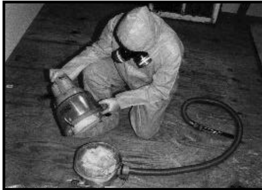
Figure 11.16a Remove the HEPA Vacuum Filters and Disassemble the Vacuum With a Plastic Sheet Underneath.
