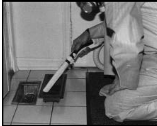
a. Vacuum and Remove Register Covers.
