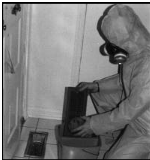
c. Wet Wash Register Covers and Replace.
