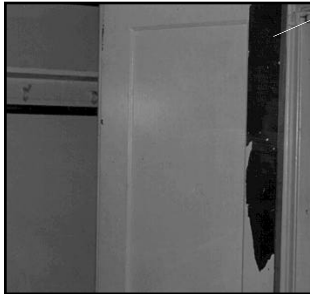
Figure 11.7 Damaged Paint on an Impact Surface.
