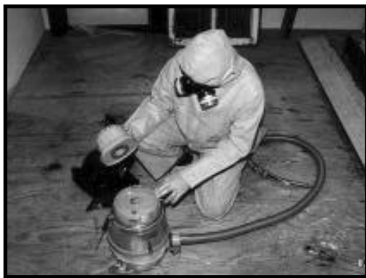
Figure 11.16f Remove and Replace HEPA Filter Assembly.
