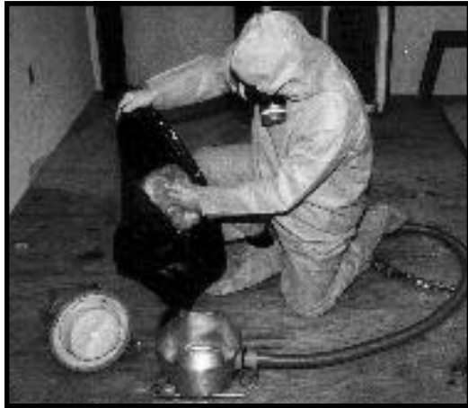
Figure 11.16d Tape Vacuum Bag Closed and Put Inside Plastic Trash Bag.
