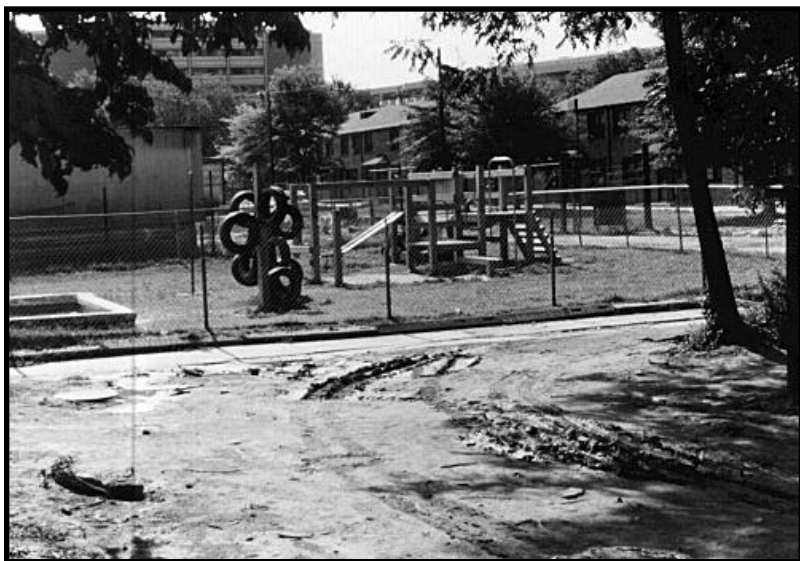
Figure 11.21b Fencing as an Interim Control for Bare Soil Hazards.
