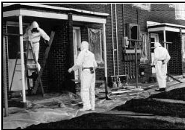
Figure 12.3b Remove and Replace Trim (exterior).
