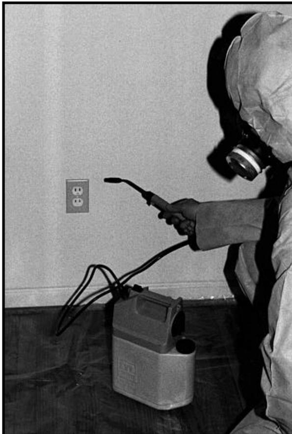
Figure 12.14 Do Not Wet Painted Surfaces Near Electrical Circuits.
