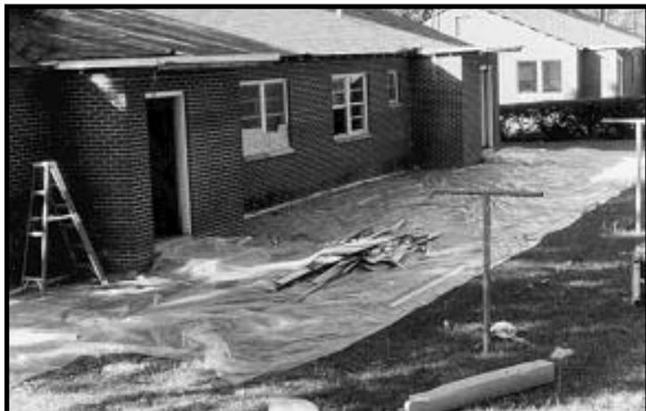
Figure 12.7a Line Walking Surfaces With Plastic.
