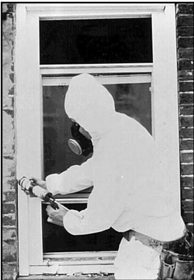
Figure 12.8b Caulk the Seams of a Window Frame Enclosure System.
