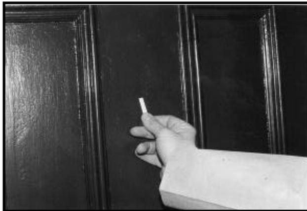
Figure 12.24 Use Litmus Paper on a Bare Stripped Surface Before Repainting.
