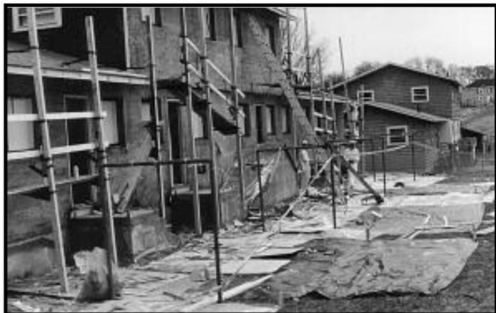
Figure 12.6 Exterior Siding Removal and Replacement.
