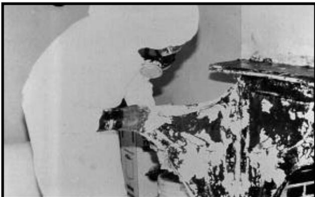
Figure 12.23a Neutralize Surfaces When Using Caustic Paint Removers.
