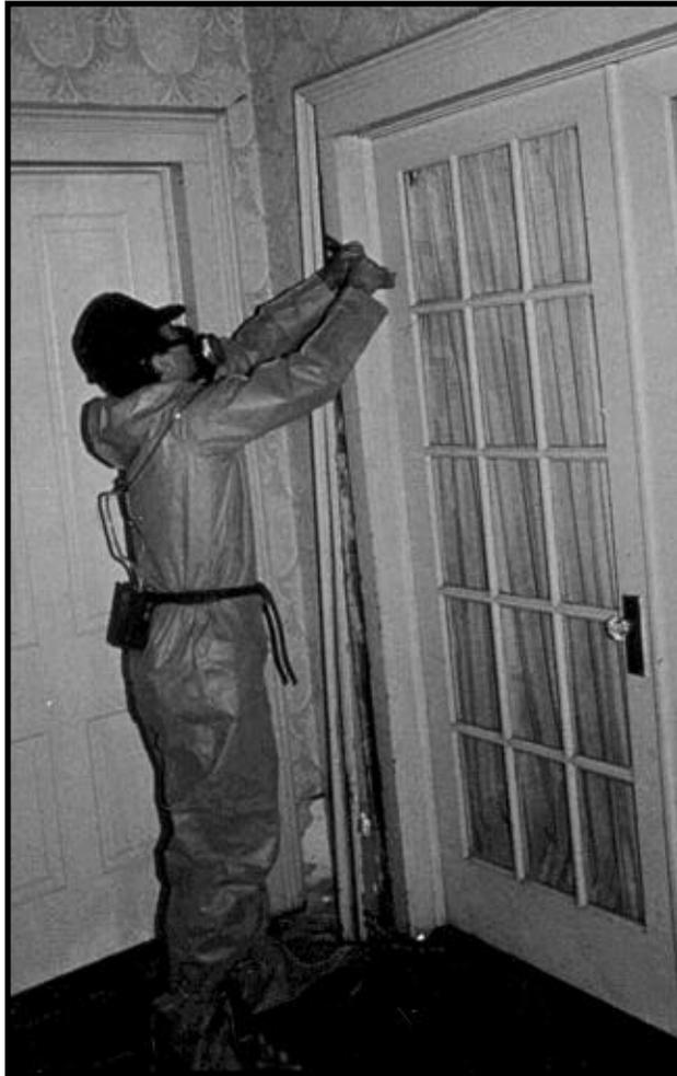
Figure 12.3a Remove and Replace Trim (interior).
