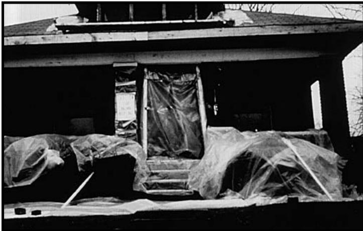
Figure 8.3b Prepare the Worksite With Plastic Sheeting (exterior).
