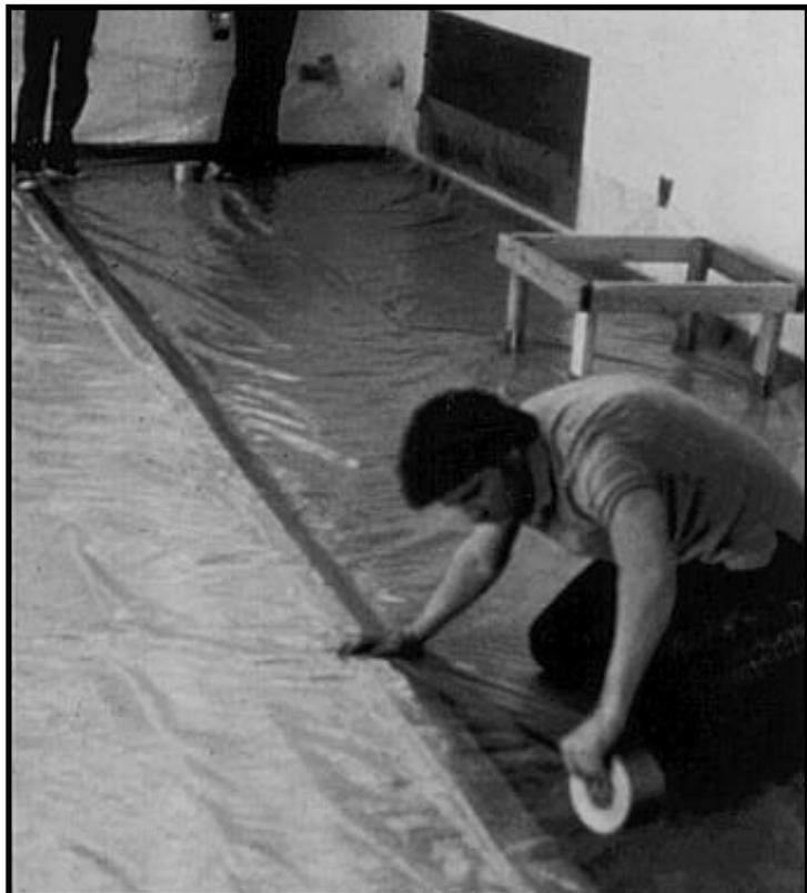
Figure 8.3a Prepare the Worksite With Plastic Sheeting (interior).
